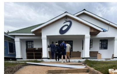
Renovation of CHOJO CAMP Facilities
