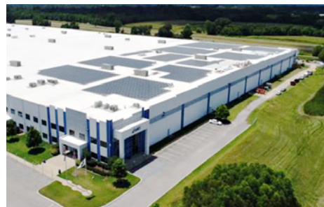
System Installation Drone View of ASICS distribution center in Byhalia, Mississippi
